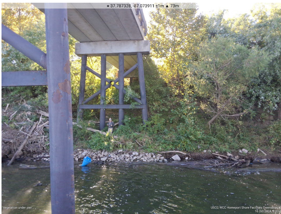
Photo 8 Vegetation under pier.
